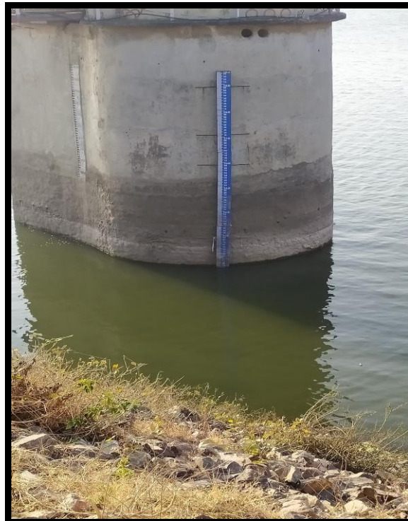
Dam Water level Scale
